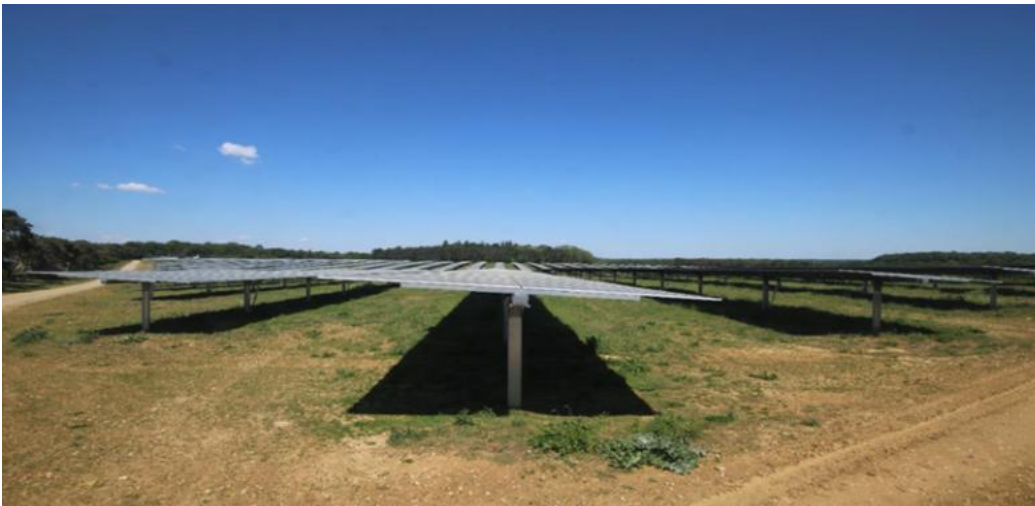
Image 4.1: Typical Single Access Tracker Panels
